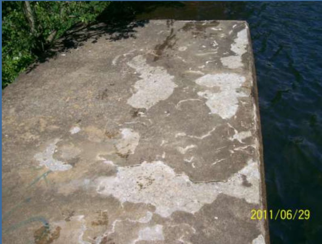
Small Scale Surface Patching
