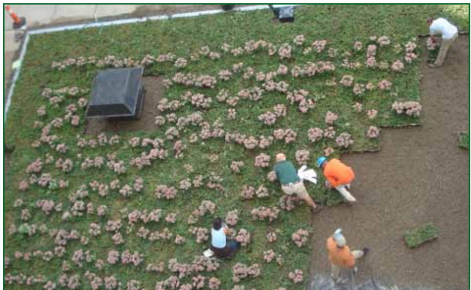
Installation of a green roof at the State Capitol.
