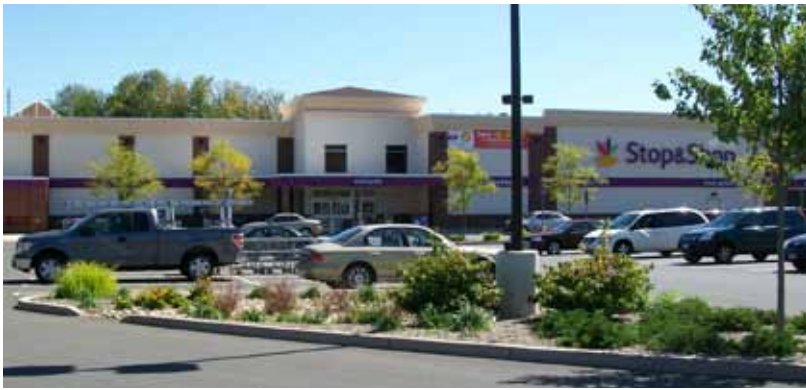
Landscaped islands filter stormwater in the Torrington Stop & Shop parking lot.
