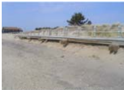
Beach Boardwalk at Hammonasset
