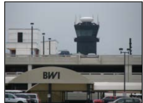
Figure 3 - Pepco Energy installed a 505 kW Solar PV Array at the BWI airport in Baltimore, MD.
